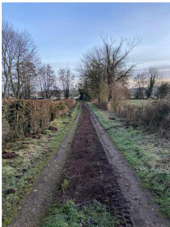
Benhall access track following improvement works
